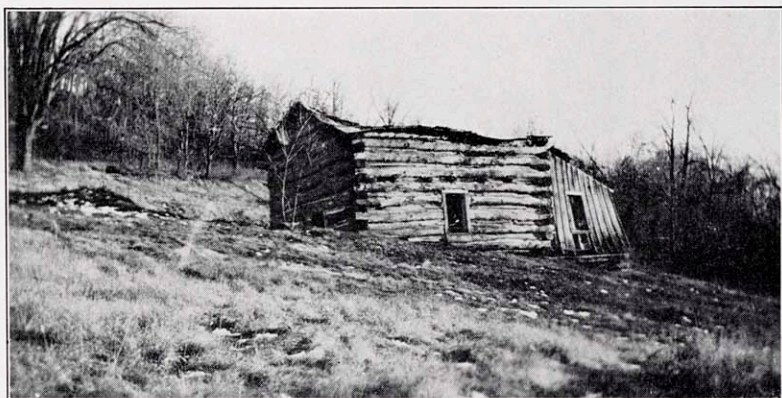
LAST OF THE MINING BUILDINGS
