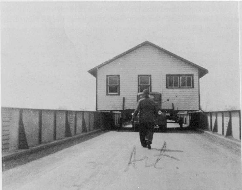
Cottage from Weigands Bay that was moved across the second Prairie du Sac bridge. It had to be jacked up higher in order to clear the bridge railings. Art Eberhart is backing up directing Jack who is driving the truck. Photo taken in 1942.
