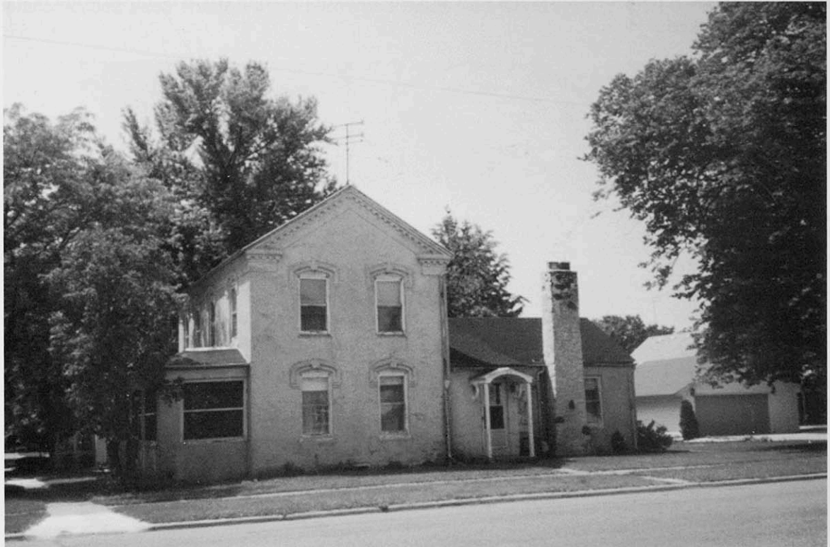
315 Washington: This home was built about 1890 by Edwin Farr. It was a cream brick home with ornate cornice and frieze and window details. It has since been covered with stucco. Other owners have been Edwin Perkins, Fred Albertus, and Roy Peterson.
