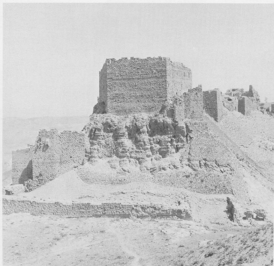
LII. a. Castle of Margat (al-Marqab) seen from the south b. tower of the castle of Kerak seen from the south
