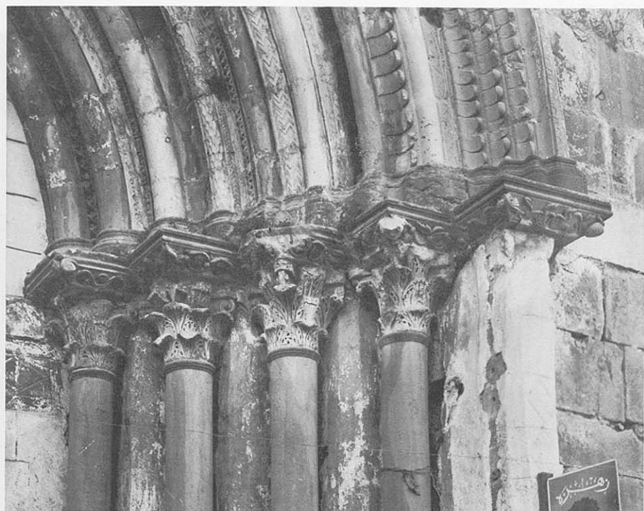
XVII. Church of the Resurrection, Nablus, now al-Jāmi' al-Kabīr: a. main door before the earthquake of 1927 b. detail, capitals on the right side of the main door
