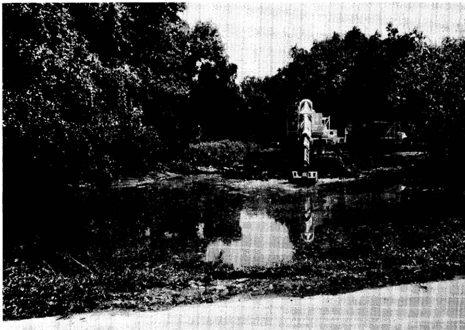
Figure 5. View of man-made pond during excavation. Gradall is removing fill road created in pond to reach perimeters of pond.
