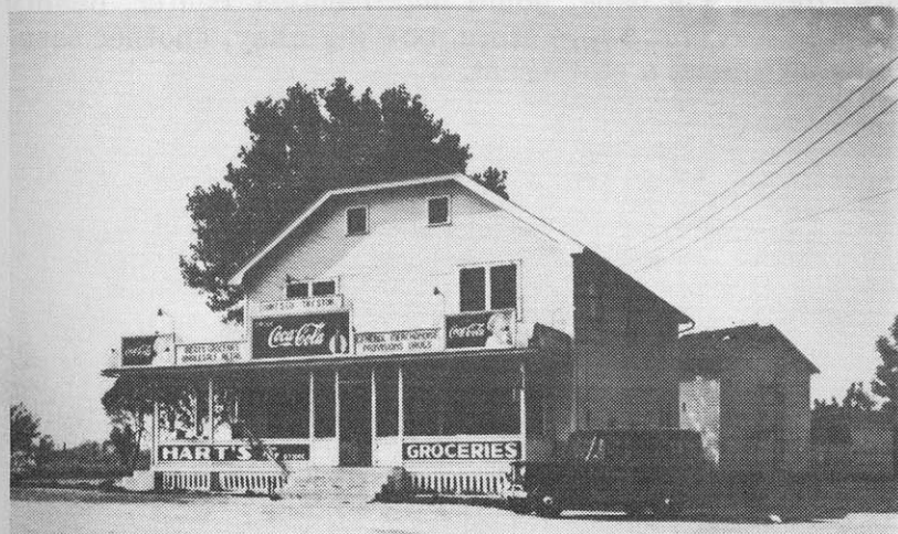
Hart's Store about 1954. Note ladder on side of ice house in rear
