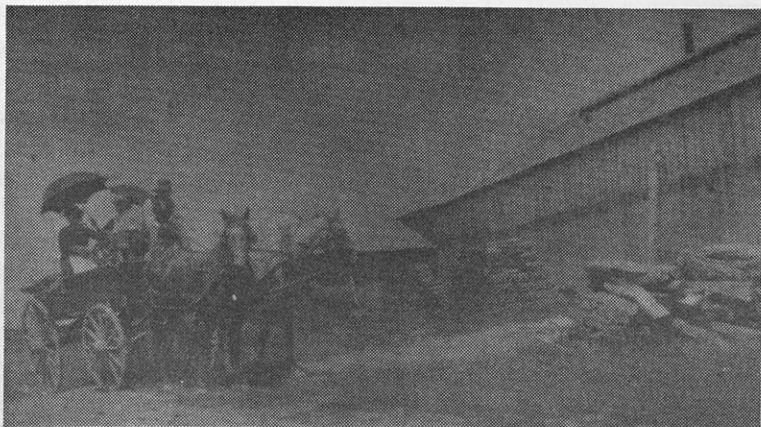
Wind Lake drainage tile factory, built about 1885 by Thompson and Eilert Friis
