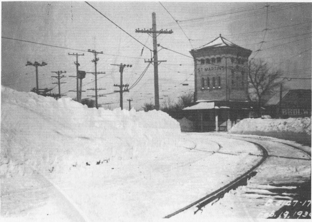
ST. MARTINS LOOKING EAST-NORTHEAST FEB. 19, 1936
