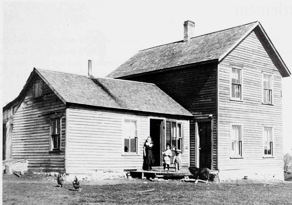
The “upright” part of the Edward and Ellen Byrne house was constructed with lumber from the 1857 St. Mary’s Catholic Church, which was dismantled after a new church was built in Oregon in 1886. The Byrne house staircase was made from the old choir loft stairs, and the bannister incorporated part of the communion rail. The Byrne house is located on Whalen Road hill, southeast of Stoner Prairie. Photo taken in 1890’s.
