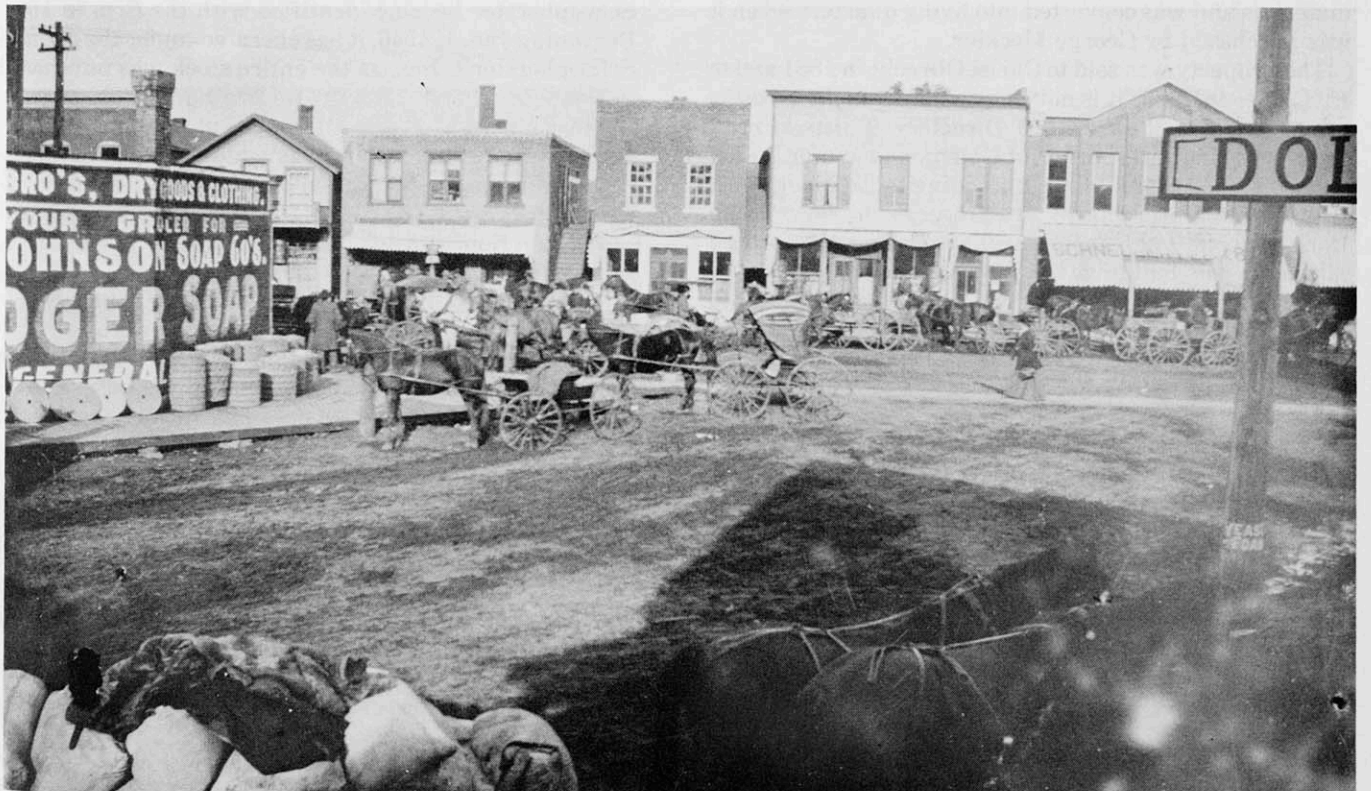
This is probably the only picture in existence taken from this angle. It is taken from the Doll building at the corner of Park Ave. and Galena St. It shows part of Conger Bros. Dry Goods and Clothing store, and the triangle on which they displayed grinding stones and bales of wire. Across the street, from left to right, part of Fey's saloon with balcony, Cumming's or
