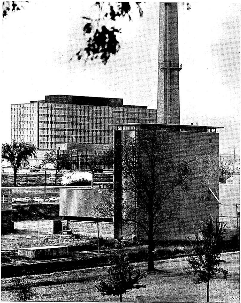
This is the new Hill Farms State Office Building complex on Madison's west side. The buildings in the foreground (on University Avenue) house the heating plant, the State Crime Laboratory, the dairy and food laboratory of the State Department of Agriculture, and the sign shop of the State Highway Commission. The 2-story building in the background contains the offices of the Departments of Agriculture, Civil Defense, Conservation, Nurses, and the Employment Relations Board. The high-rise office building behind it (it fronts on Sheboygan Avenue) is the new home of the Departments of Banking, Insurance, Motor Vehicles, the Industrial Commission, and the Public Service Commission.
