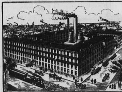
(View of Works.)
