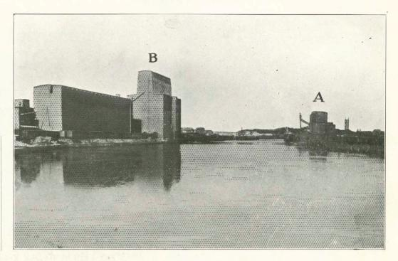
THE grain elevators "A" and "B" are owned and operated by Bartlett Frazier Co., and are among the largest in the country, having a combined capacity of 2,500,000 bushels.
