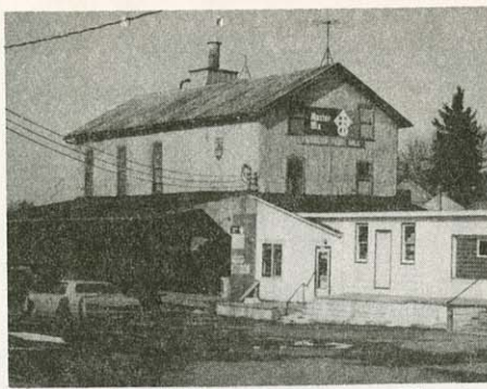
Fessler's Feed Mill and Elevator. Elevator built in 1901.
