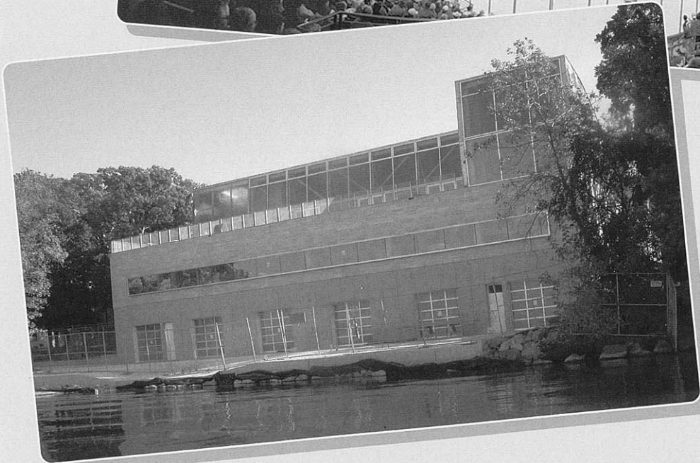
Left: Wisconsin's rowing programs look forward to a new crew house, which will open in December, 2004.
