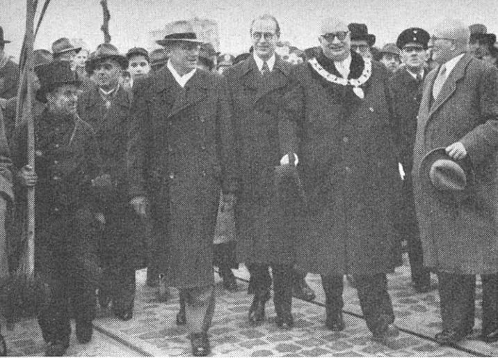
Officials presiding at recent "Peace Bridge" dedication ceremonies in Frankfurt are escorted to southern bank of Main River by traditional chimney sweep, symbol of good luck. The new span is largest of its type in Western Germany. Next to sweep are US State Commissioner for Hesse James R. Newman, Hesse Minister-President Georg August Zinn and Frankfurt's Mayor Walter Kolb. (PRB OLCH photo)
