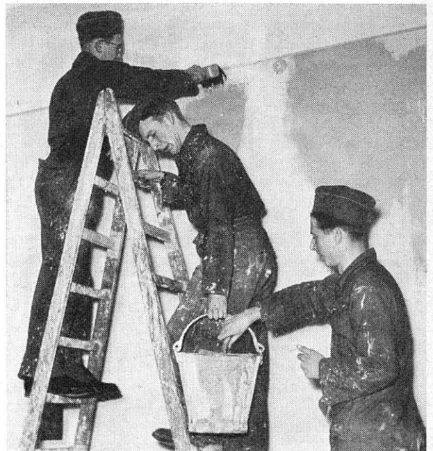
It's questionable where more paint is being applied: on walls or on dungarees of young volunteer workers making last minute preparations for recent opening of a new Neighborhood Home in Zehlendorf, Berlin. However, their efforts produced an attractive and much needed center which was partly financed by grant of DM 160,000 from HICOG Special Projects Fund. (PRB BE-HICOG photo)
