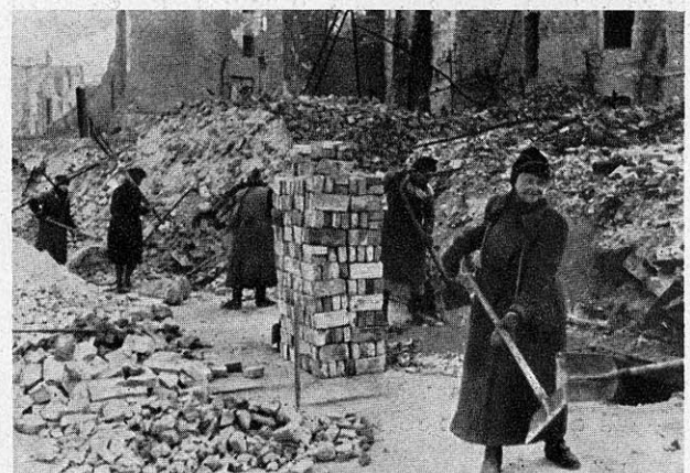
WPA-like projects, sponsored by the Magistrat, helped absorb blockade unemployment in Western Berlin and clear some of the mountainous debris from the city's ruins.
