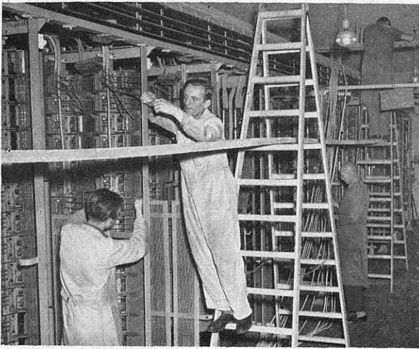
Workmen repairing one of the nine telephone exchanges in the U.S. Sector damaged by war-time bombing.
